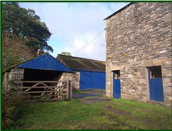
Workshops 1,2, store and barn from the driveway
